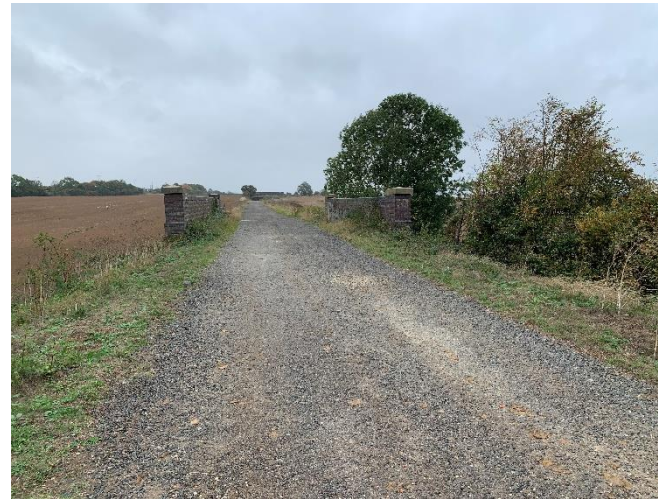
Fig 71 and 72 West and East approaches to the existing Knuston Brook bridge.
