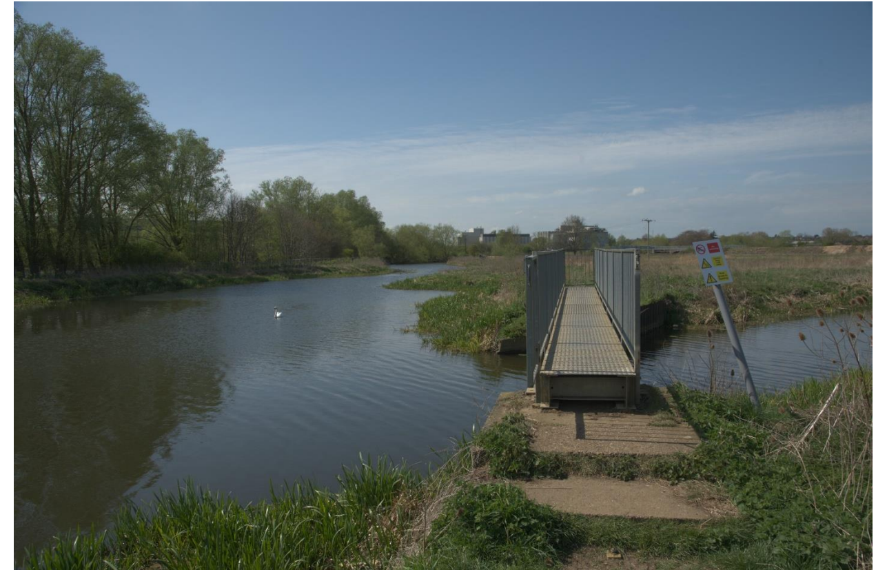
Fig 01 Existing bridge over the creek on the River Nene, inaccessible for many potential users.
