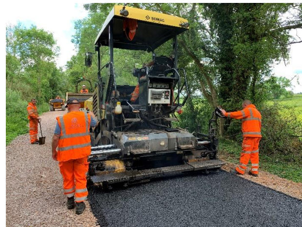
Figure 8: Smooth, tarmac surface, accessible for all non-motorised users
