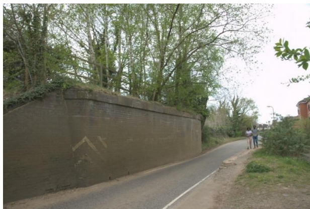
Fig 28 Removing the bridge abutment and creating a sinuous ramp within the railway formation may retain the route in one landowner but risks greater ecological impact.
