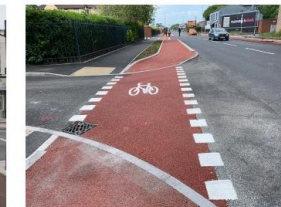
Priority to cyclists can be provided at side roads even in industrial areas using coloured surfaces and markings.
