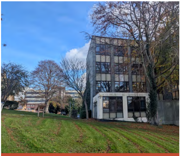
Council Offices on Tithe Barn Road
