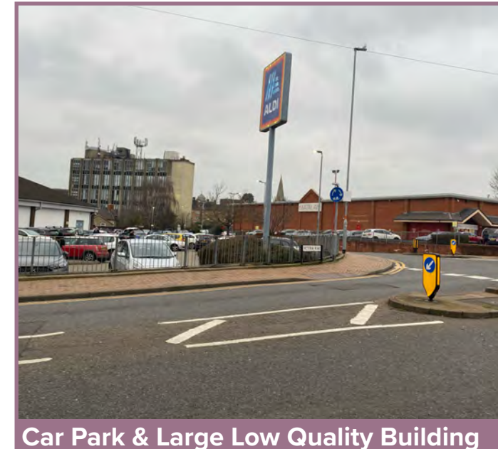
Car Park & Large Low Quality Building
