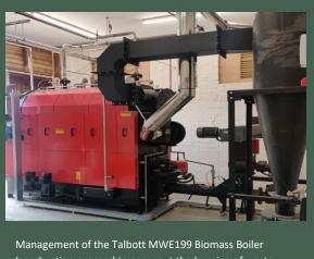
Management of the Talbott MWE199 Biomass Boiler 'combustion process' to carry out the burning of waste wood as prescribed by EPR Section 6.6 PGN 6/02(12).
