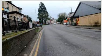
Pinch point outside Sainsbury's due to level differences. Remove the right turn pockets to accommodate a continuous segregated route.
