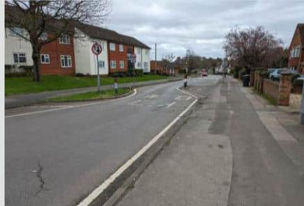
One-way segregated westbound (uphill) cycleway between Northampton Road and Croyland Park. Insufficient width along Croyland Road to provide a two-way segregated route. Provide cycle bypasses at existing chicanes to give priority to cyclists. Reduce speed limit to 20mph.
