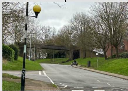
Pinch point on Nest Farm Road due to the pedestrian overbridge. It is proposed that the segregated route will connect to the pedestrian overbridge and down the other side due to the width constraints under the bridge.
