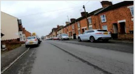
Several pinch points along this section caused by on street parking outside terraced properties and outside of Newton Road Community Primary School. The on-street parking means that there is insufficient width through here to accommodate a segregated cycleway, so an alternative quiet mixed street route is proposed.
