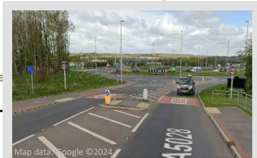
Upgrade existing uncontrolled crossing to a signal-controlled pedestrian and cyclist crossing to improve access on/ off the proposed A6 segregated cycleway.
