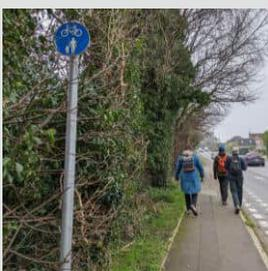
Widen existing narrow shared use path to a two-way segregated cycleway on the eastern side of the carriageway. Right turn pockets to be removed to accommodate the segregated cycleway.
