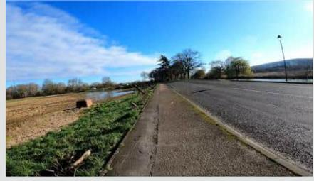
Two-way segregated cycleway along the western side of Embankment. Remove hatching and right turn pockets to accommodate the cycleway. Some land take may be required.
