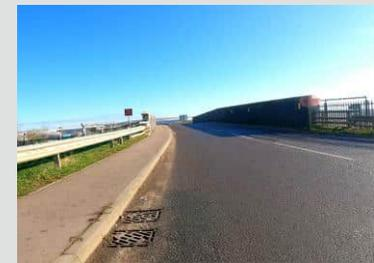
Pinch point over the railway bridge. Cyclists will have to rejoin the carriageway here. There is potential to incorporate some traffic signals over the bridge to give cyclists priority.
