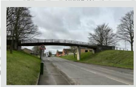
Two-way segregated cycleway diverted off the carriageway for a short section due to a pinch point caused by a pedestrian bridge over Queensway.
